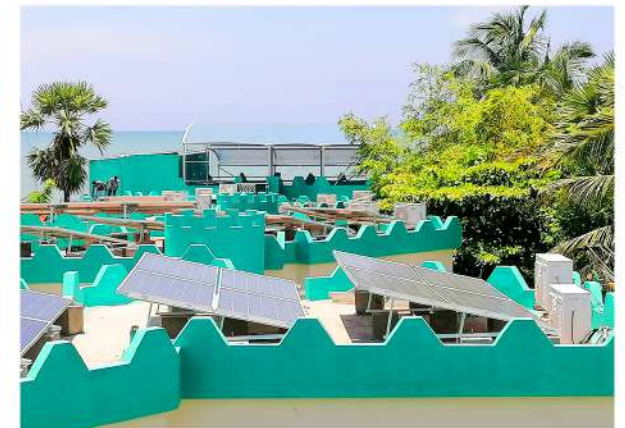
36 KW - Lamel Cove Beach Resort Auroville, Tamilnadu
