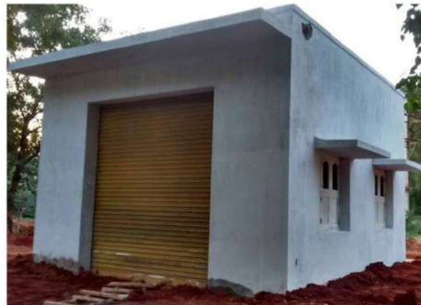
Jipmer Campus - Pipe line, Water Treatment plant
